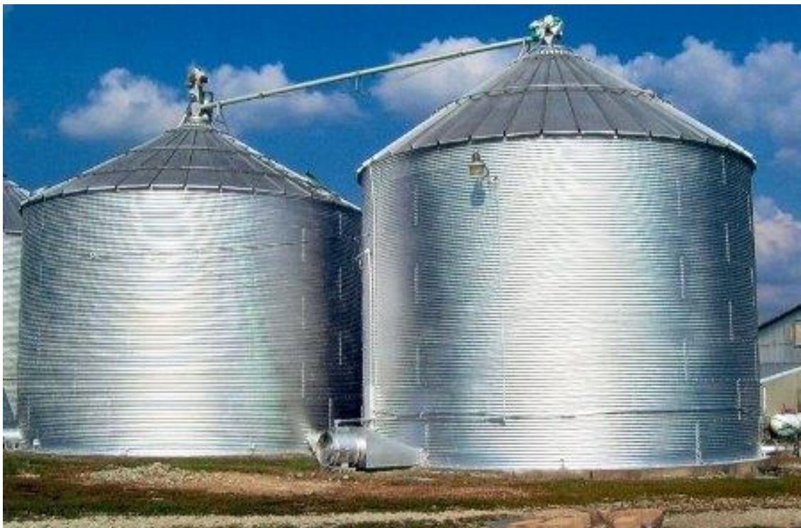
Figure: Bean storage steel bins with monitored air flow at the bottom.
