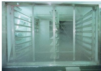
Air Blast Freezer
