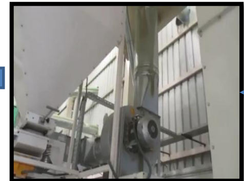
Cleaning with centrifugal blower
